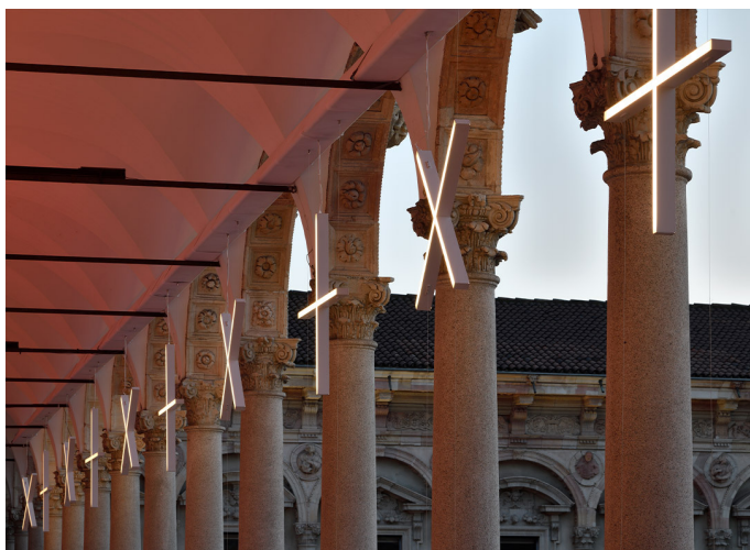
Tetras - Skidmore, Owings & Merrill (SOM)
