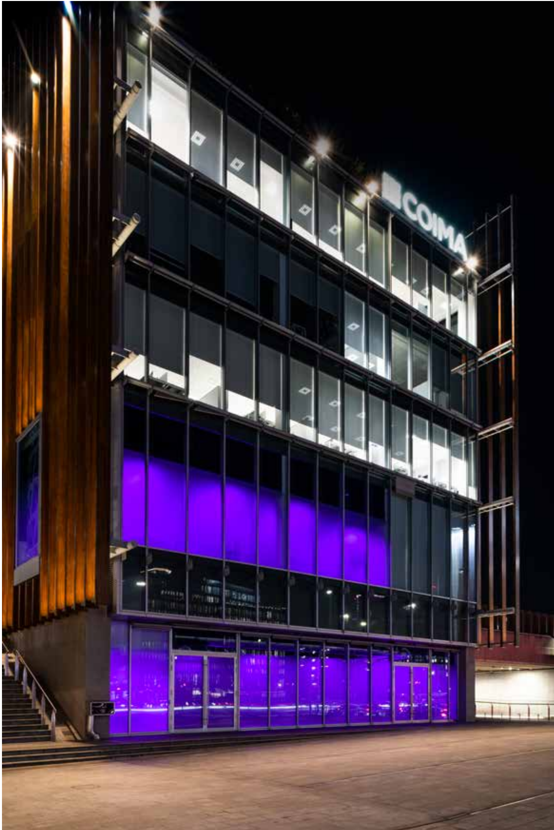
INTEGRALIS® installation HabiSmart by COIMA - Milan, Italy
