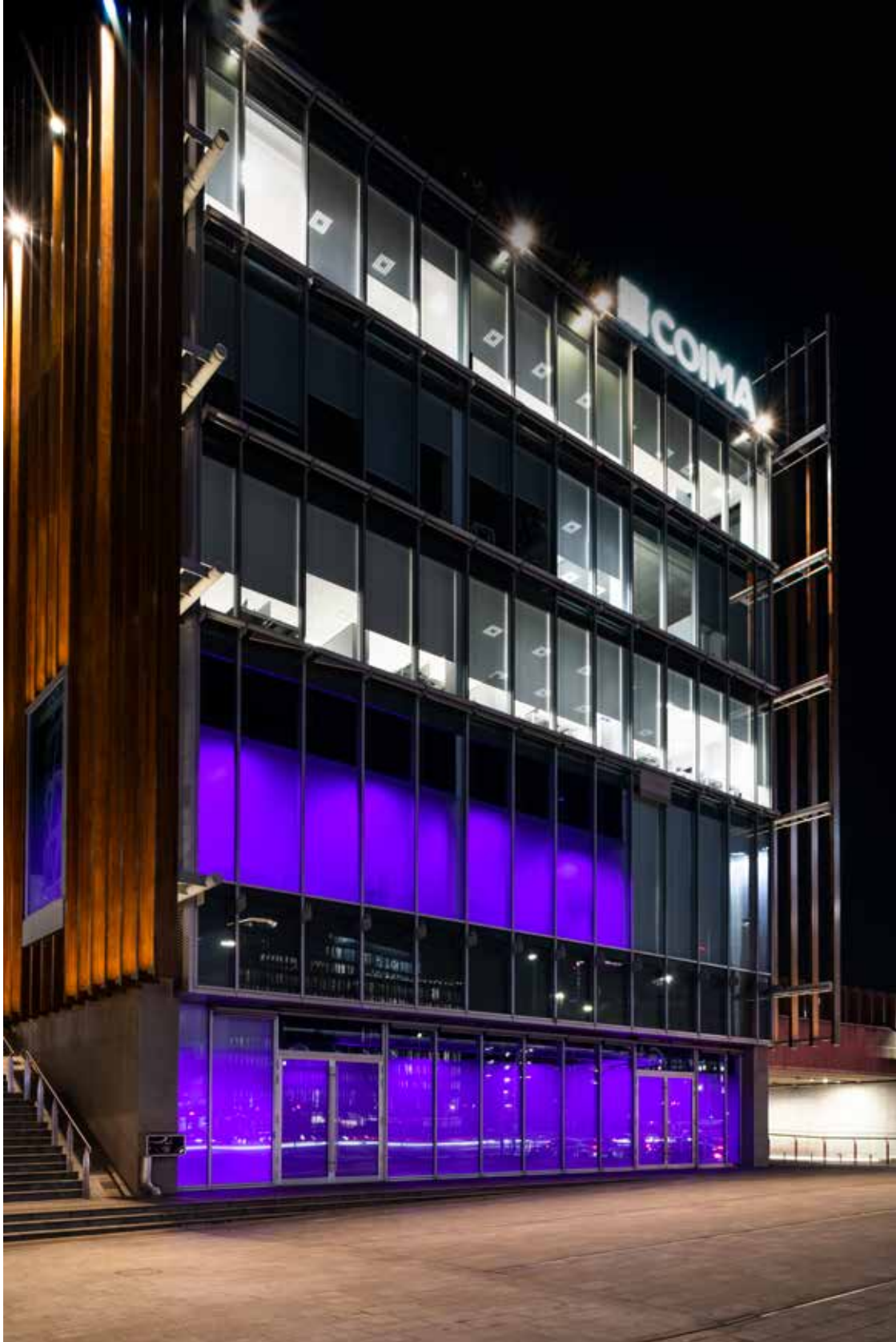
INTEGRALIS® installation HabiSmart by COIMA - Milan, Italy
